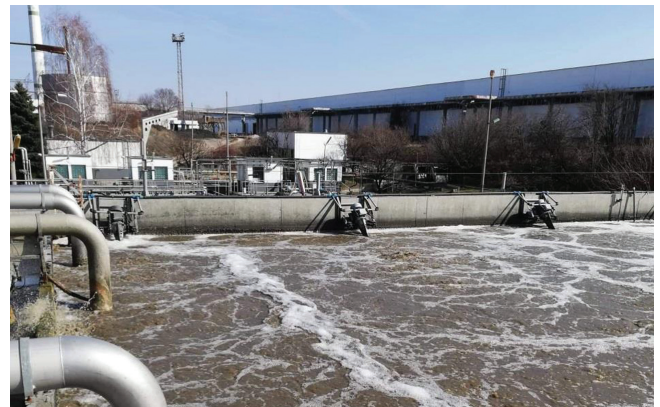
OxyStar® Aspirating Aerators Mounted Directly to Basin Wall
