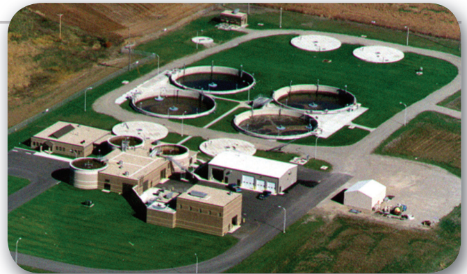
Aerial view of Clear Lake showing four AquaSBR ® basins.
