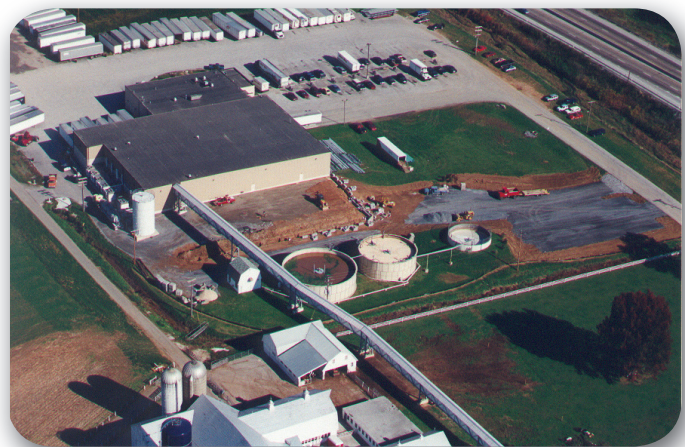
Aerial view of the Rutter's Dairy treatment plant.
