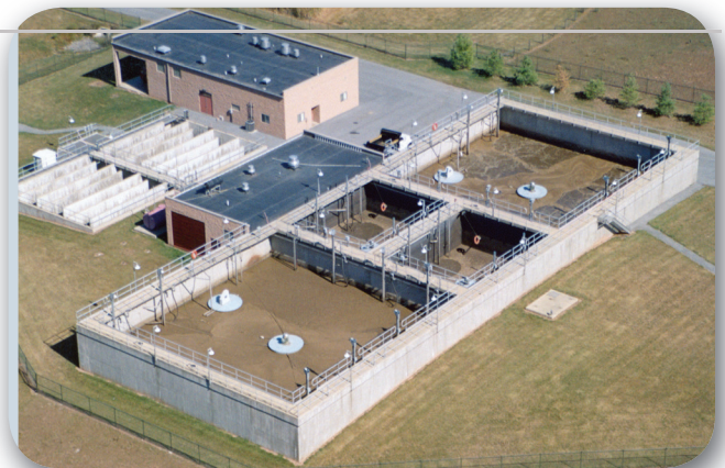
Close up of the AquaDDM ® mixer and Aqua-Aerobic Electric Actuated Decanter in one of the 2 AquaSBR ® basins.
