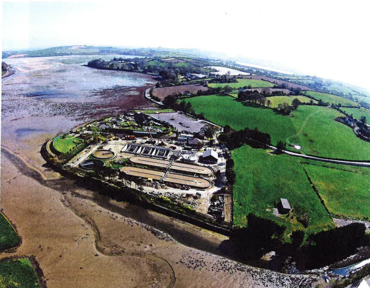
An aerial view of Clonakilty Wastewater Treatment Plant, County Cork.
