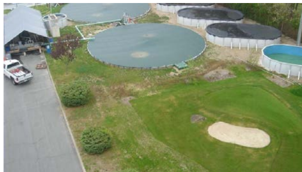
Figure 1: Pilot Plant Building (upper left) and Replica Golf Course Hole (lower left)
