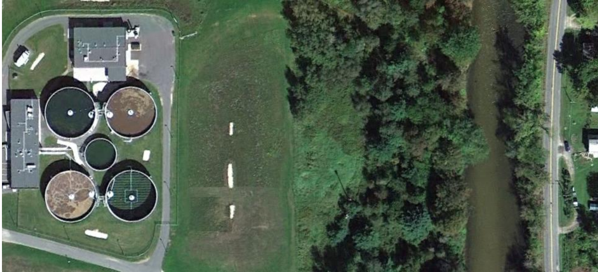
Figure 2. Aerial view of the Lee, MA WWTF and the Housatonic River.
