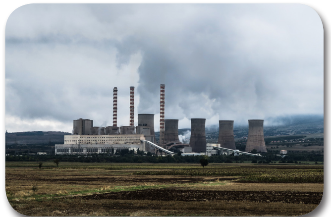
Industrial Power Plant Skyline
