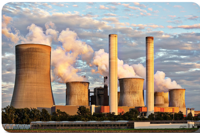
Power Plant Industrial Chimney
