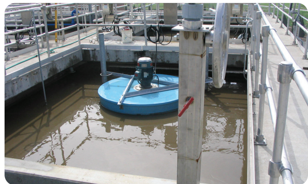
AquaDDM ® mixer with restrained mooring.
