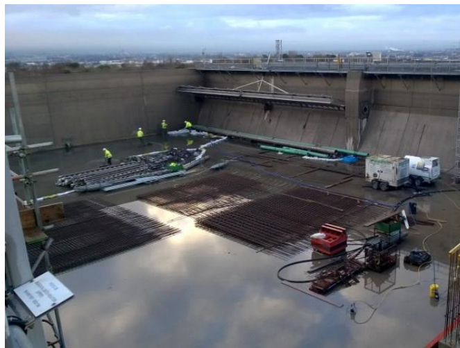
Figure 13: Retrofit Full Scale Installation Dublin Ringsend, Ireland
