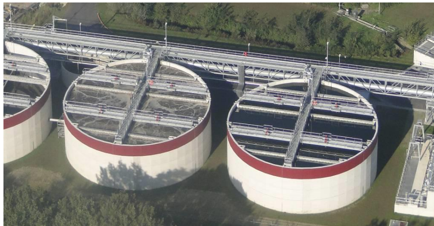
Figure 9: Full Scale Installation Epe, NL
