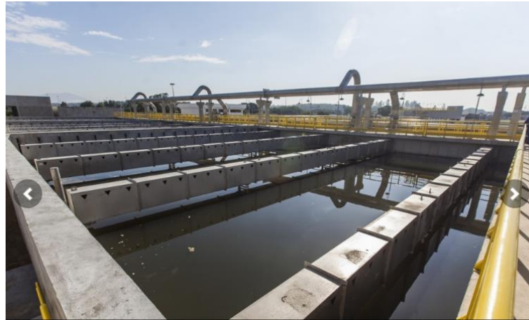
Figure 12: Full Scale Installation Deodoro, Brazil
