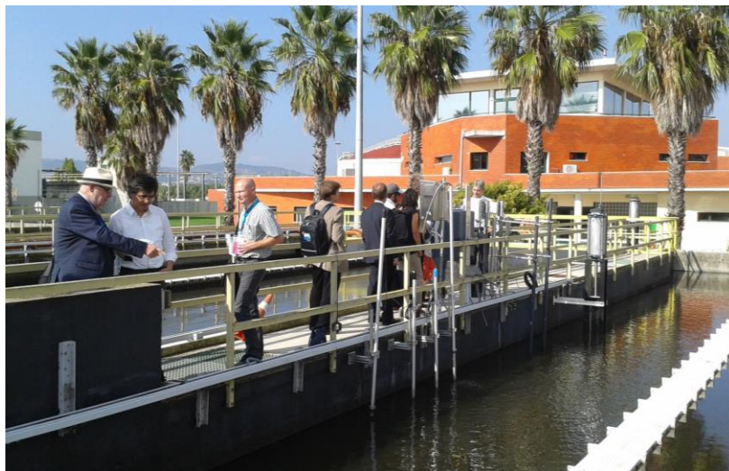
Figure 11: Full Scale Installation Frielas, Portugal
