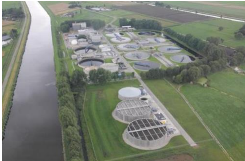
Figure 10: Full Scale Installation Gammerwolde, NL
