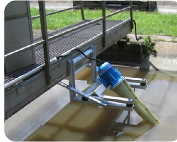
Fix mounted TurboStar® in an oxidation ditch
