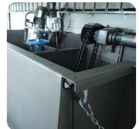
External view of the compact filter tank using OptiFiber® pile cloth media.
