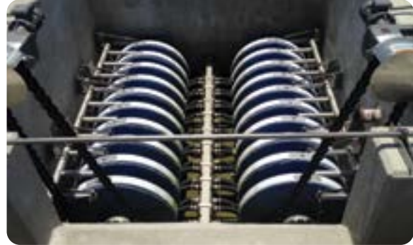
The modular design of the Aqua MiniDisk® filter retrofits neatly into existing 9 ft. (2.74 m) wide concrete traveling bridge filter basins, providing more than two times the hydraulic capacity of the original sand filters.
