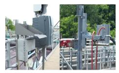
The IntelliPro system is a PC based process control system that receives, interprets and proactively responds to the loading variation in the biological process.
