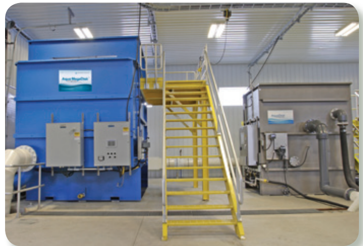
Aqua MegaDisk™ filter (left) next to an AquaDisk® filter (right).
