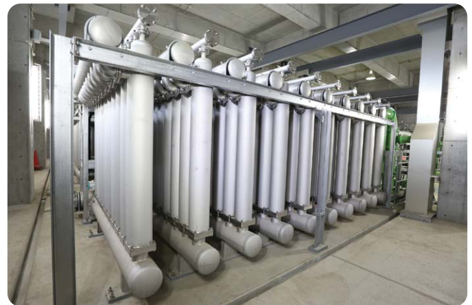
Aqua MultiBore ® C-Series Typical Installation
