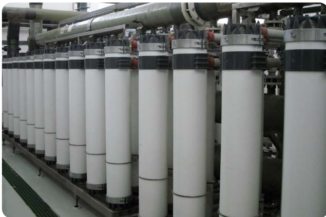
Aqua MultiBore ® Polymeric Membrane Installation
