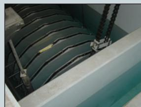
The AquaDisk filter uses pile cloth media consisting of abundant individual fibers that provide solids storage depth. The pile media permits clarified influent to
