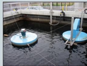
The AquaSBR sequencing batch reactor is an activated sludge process in which all phases of treatment are accomplished within a single reactor.
