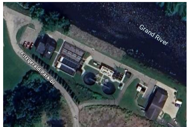
Figure 1. Existing Grand Ledge WWTP
