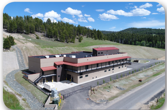
Basin Creek Water Treatment Plant - Butte, MT
