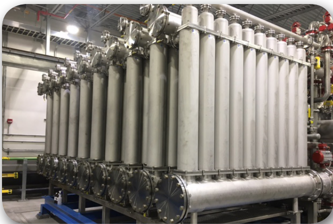
Primary Ceramic Membrane Train - Butte, MT
