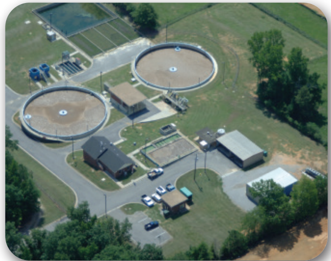
Aerial of the 2-basin AquaSBR ® system with adjacent (2) 6-disk AquaDisk ® filters
