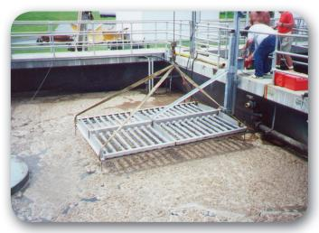
The new fine-bubble assembly on the existing track is being lowered into the basin.
