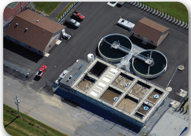
The AquaPASS® system at Salisbury Township WWTP is located next to a recreational park (shown left) and several Amish farms.
